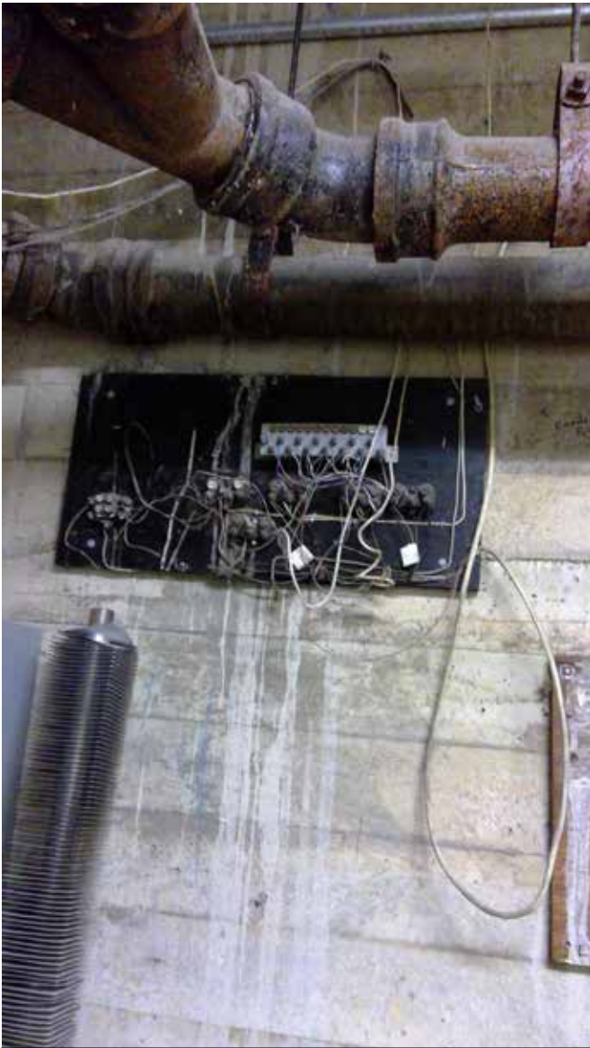
Antiquated Water Pump Control System
