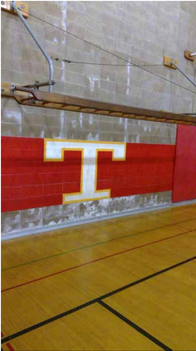
Water Intrusion at Gym Wall
